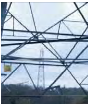
View from Woodington towards Wellow Mill.
