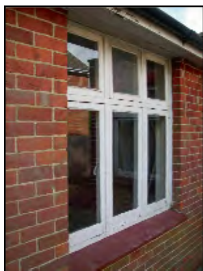
Softwood window with fixed and opening sashes and vent lights
