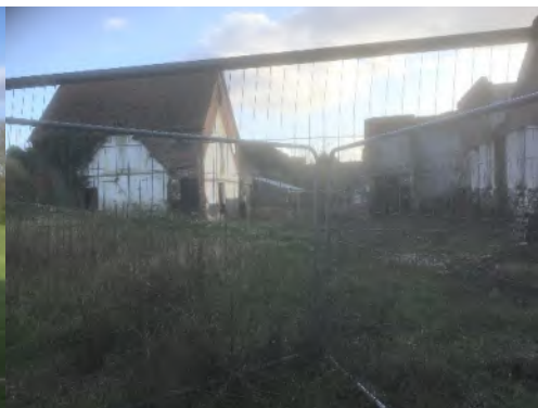
Figure 137: Derelict farm buildings
